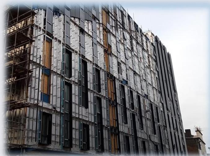
The scheme has been halted for several years due to issues surrounding development funding. Now under new ownership, the design and construction have been scrutinised and it appears that a combustible insulation may have been used in the original cladding system. This has since been replaced and new work completed using URSA's specialist product.
