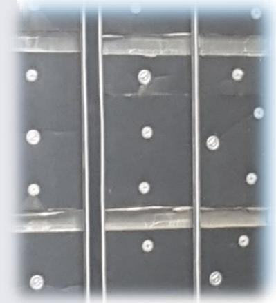
Ian added: "URSA Façade N35 is totally non-combustible, Euroclass A1, so doesn't add any fire load to the building or prejudice the overall fire performance of the wall. The presence of the ventilated cavity behind the cladding system means that cavity barriers are required to prevent the spread of fire and/or smoke. This is a unique and highly effective product that we are seeing specified increasingly across UK and European sites."
